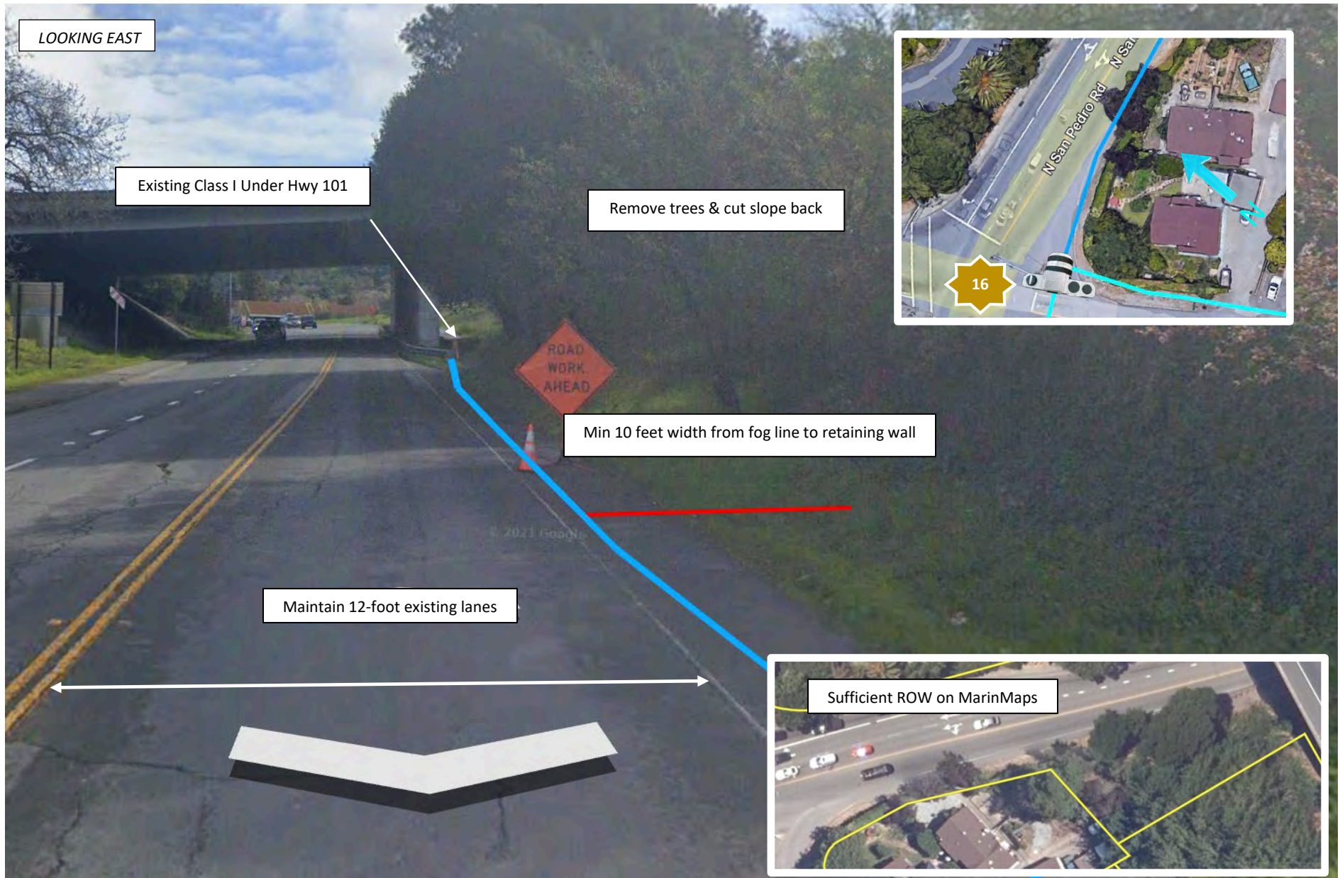
Exhibit 16 – Light Blue Segment – Looking East on North San Pedro at Merrydale
