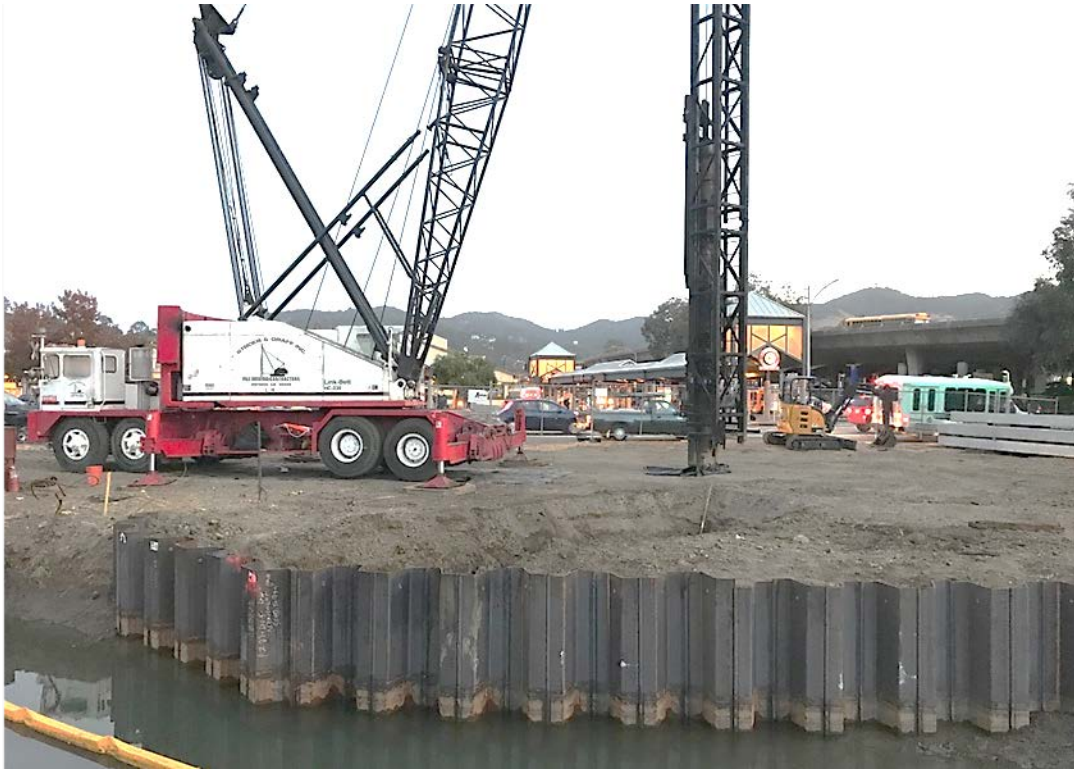
Completed sheet pile installation at the north end of San Rafael Creek Bridge
