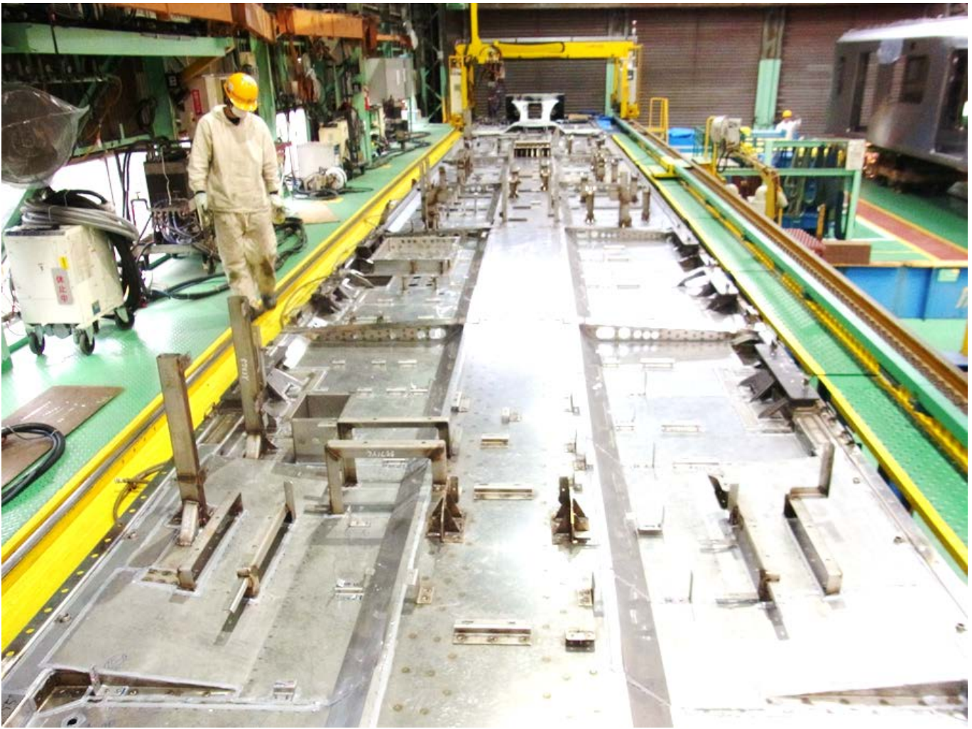
Car No.115 bottom of underframe
