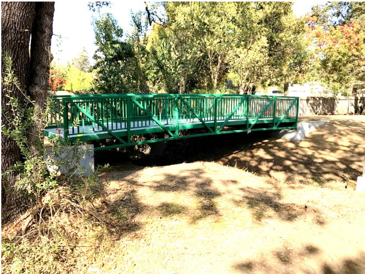
Pedestrian pathway bridge south of the Civic Center Station has been installed.
