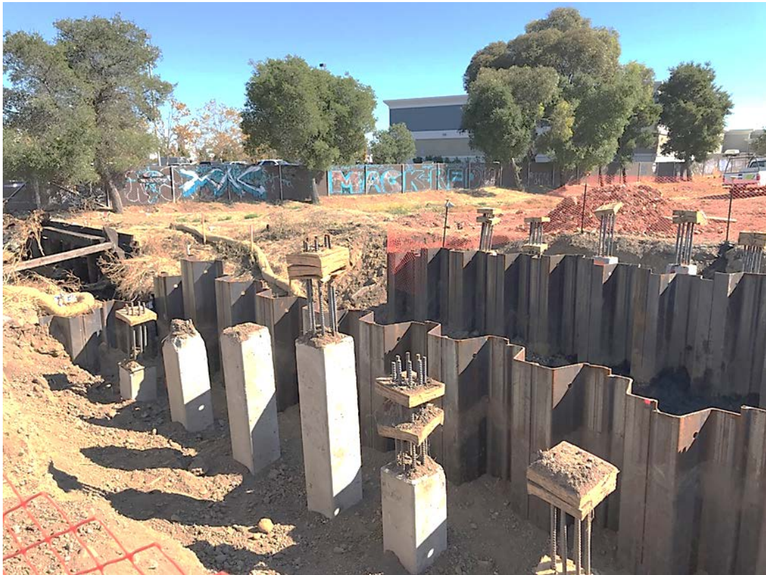
Concrete and sheet piles installed at Unnamed Channel Bridge
