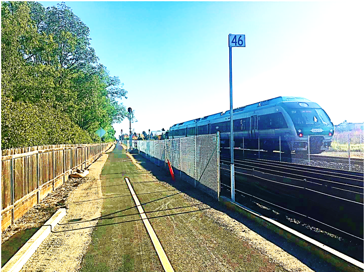
Completed pathway south of the Cotati Station.
