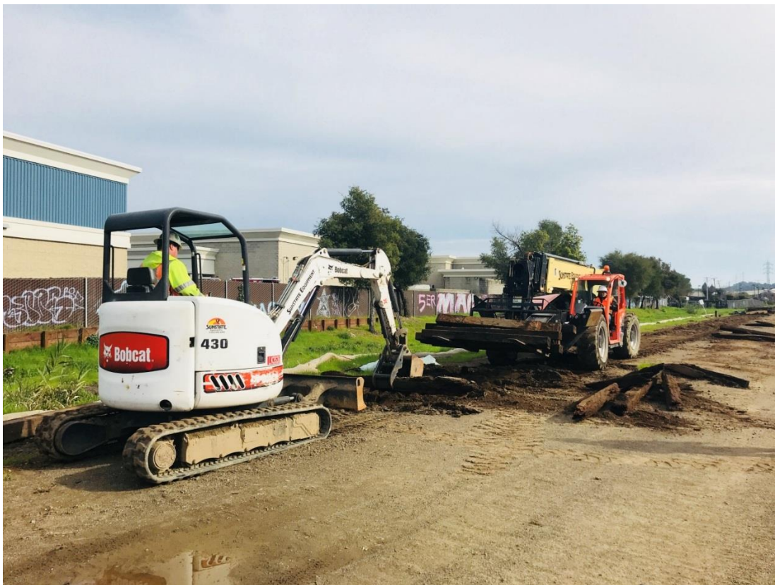
Tie removal north of Andersen Drive
