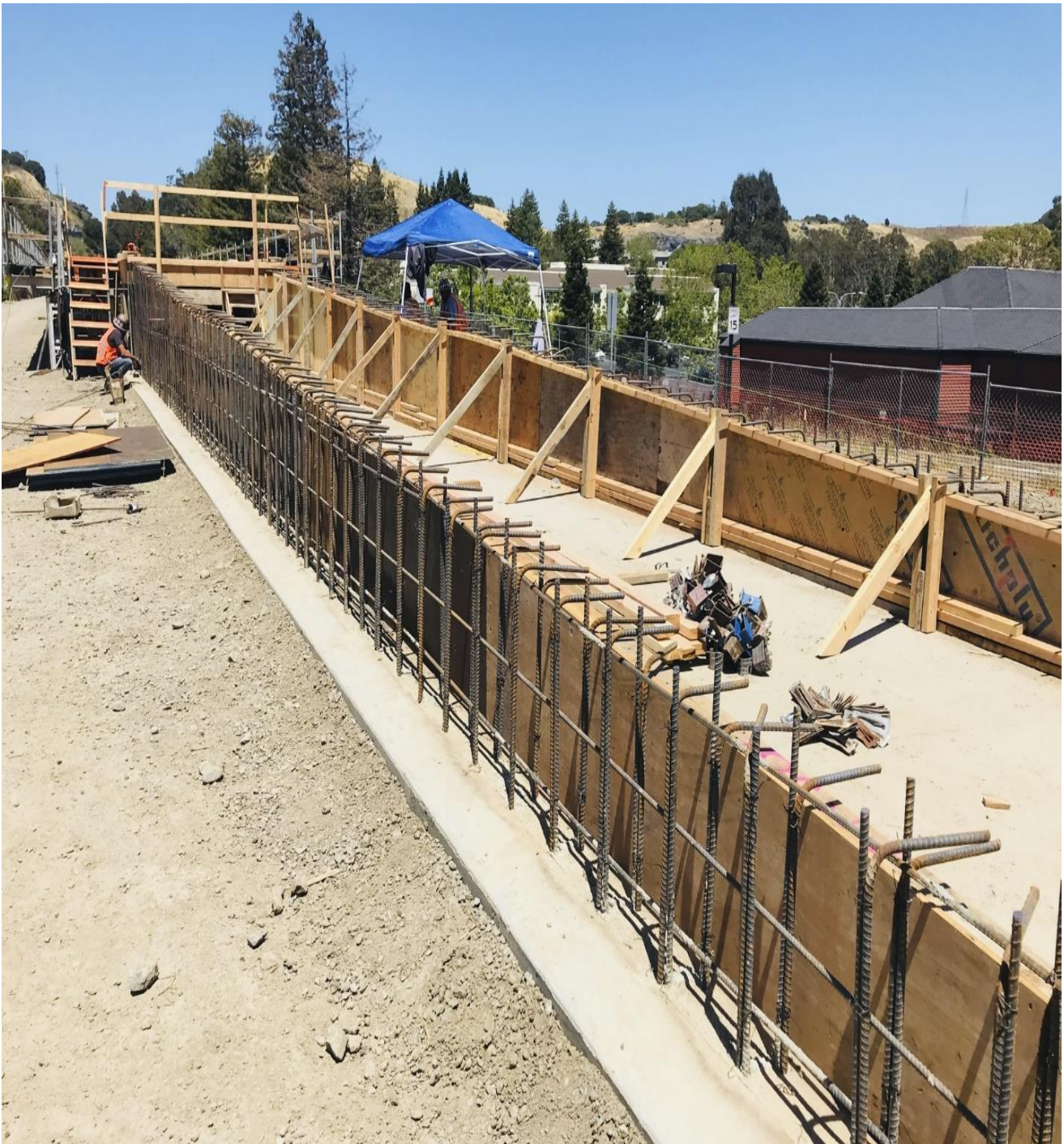
Larkspur Station Platform Ramp – concrete formwork
