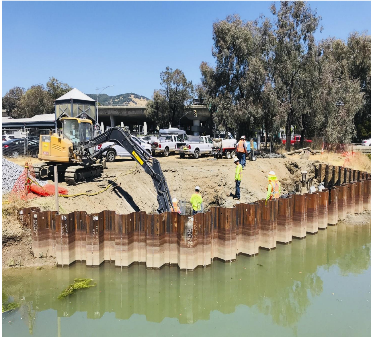
San Rafael Creek Bridge – foundation construction
