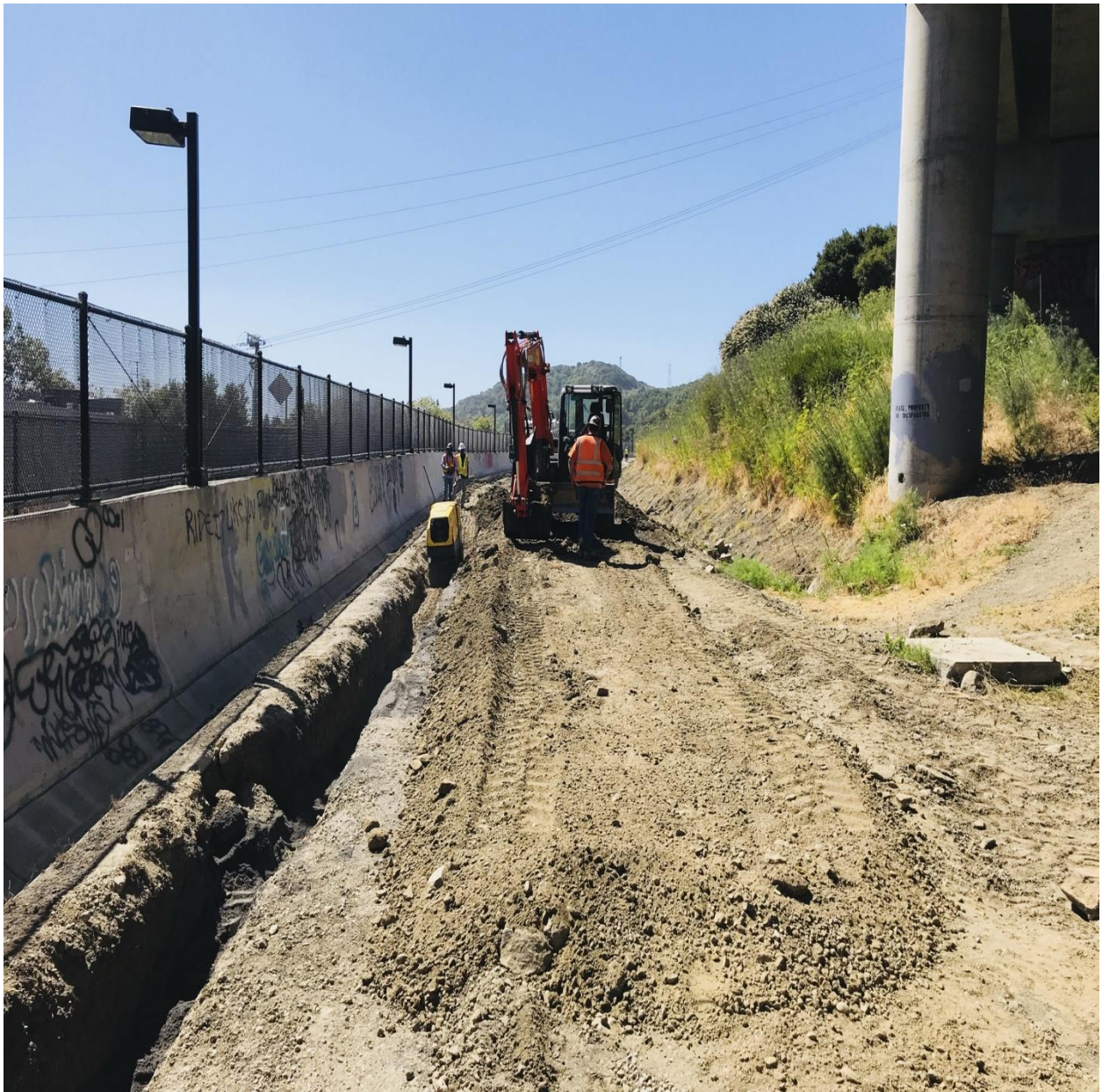
Excavation for utilities from near the Auburn Street Bridge
