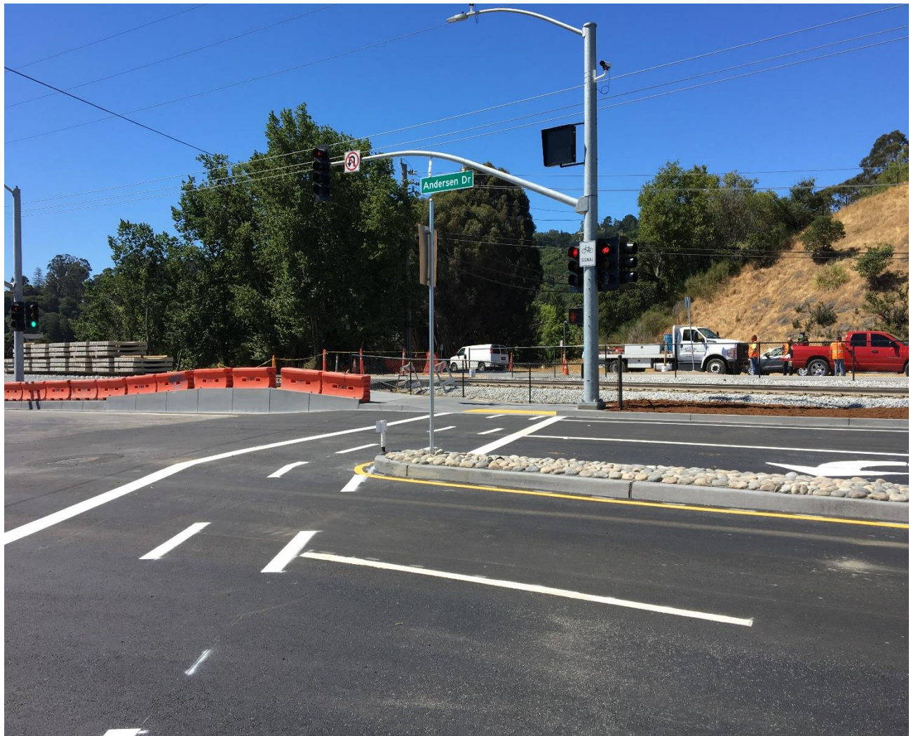
Andersen Drive At-Grade Crossing
