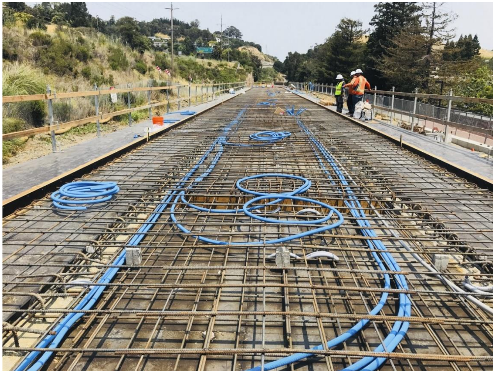
Larkspur Station Platform Construction
