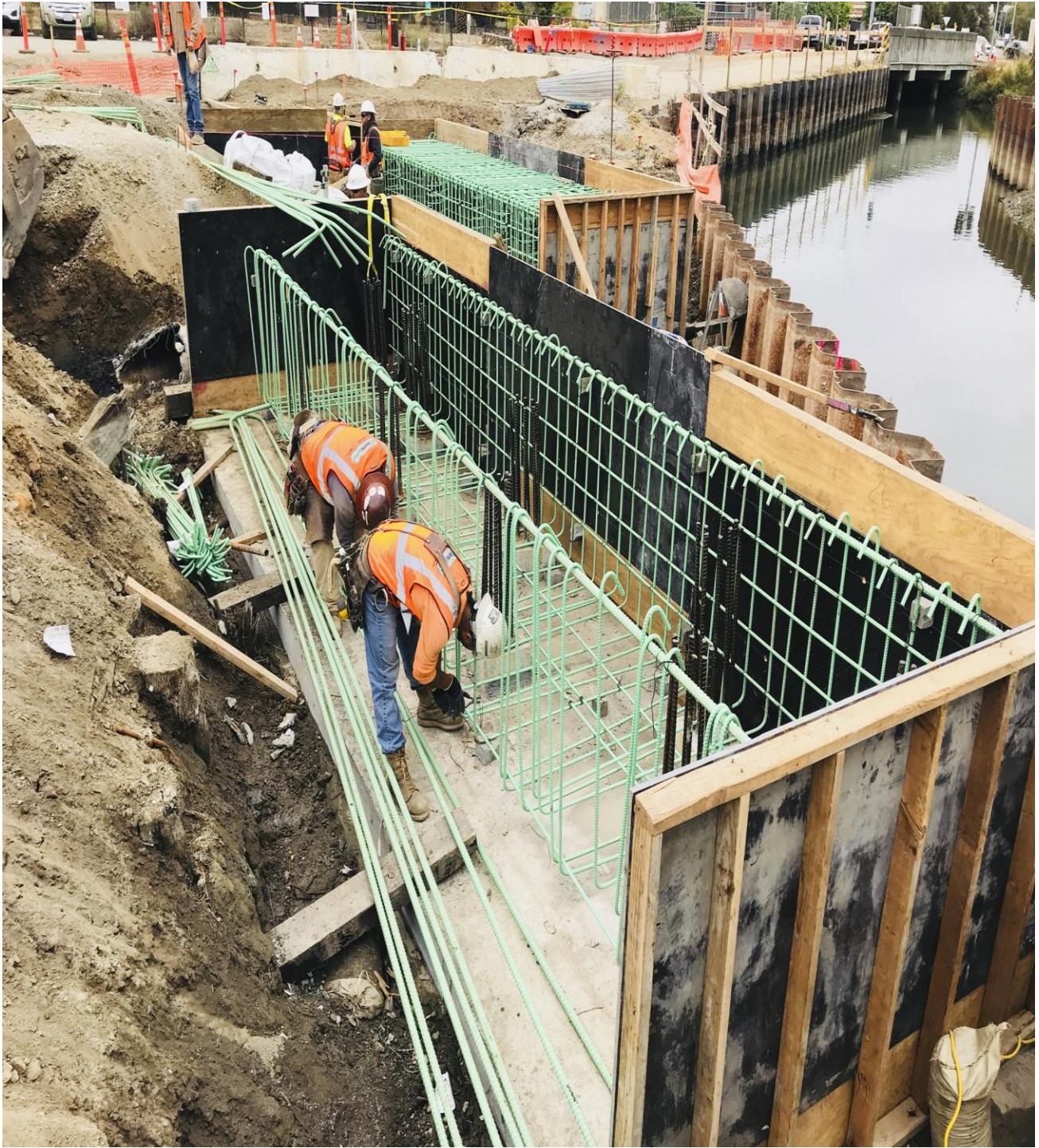
San Rafael Creek Bridge Rebar Instalation for the bridge foundation
