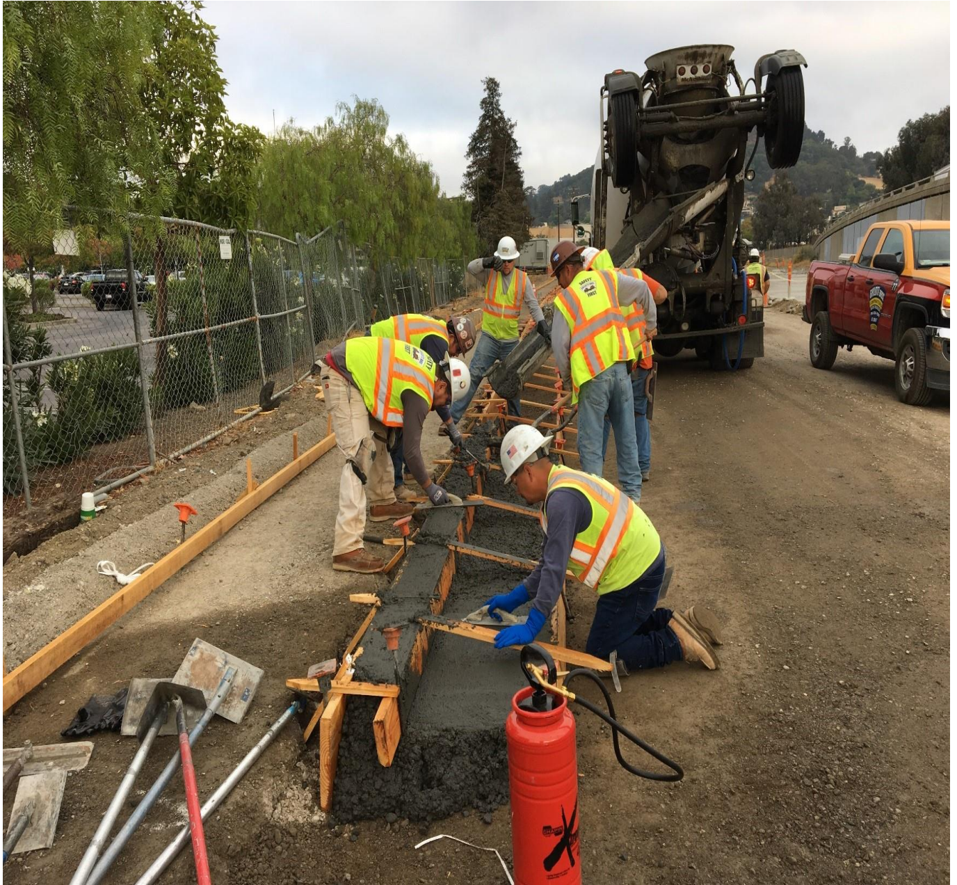
Francisco Blvd West curb and sidewalk construction
