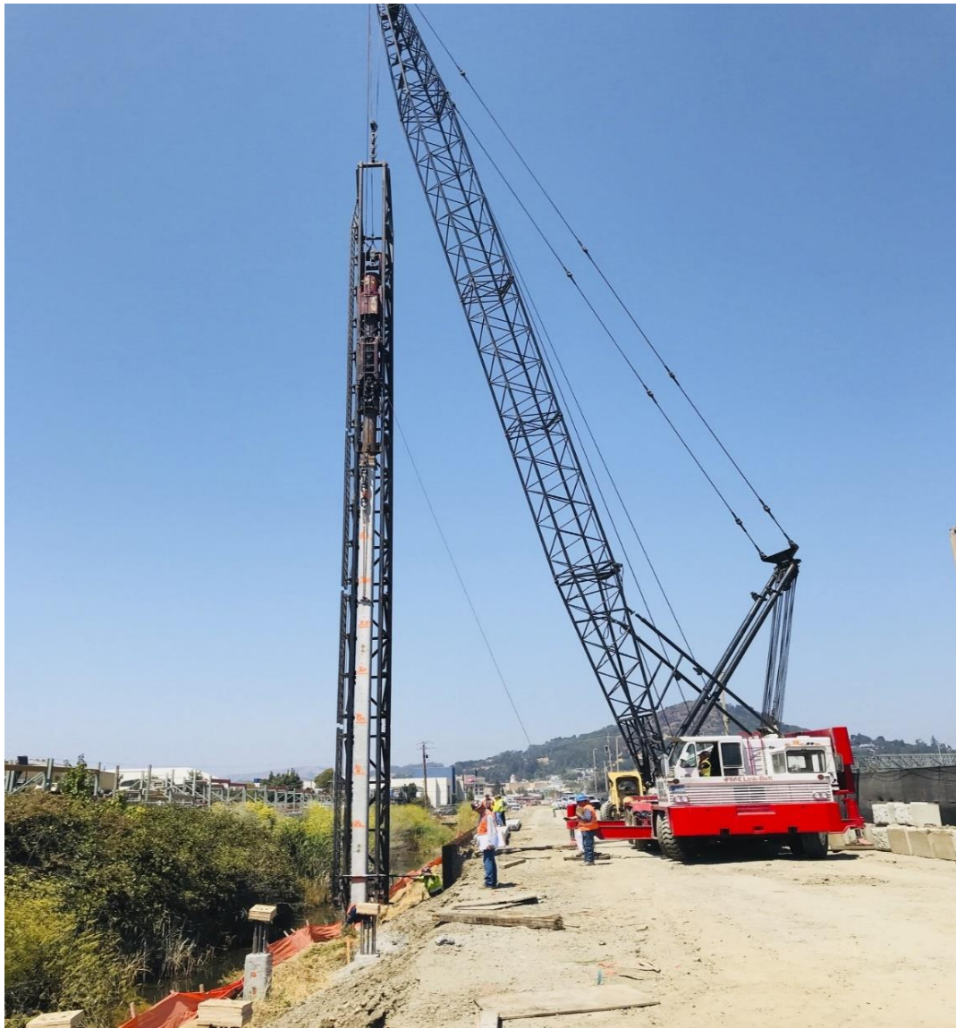
Multi Use Pathway, Sheet Pile Driving
