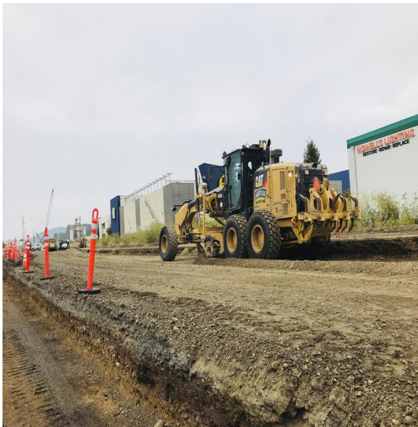
Francisco Blvd West roadway grading
