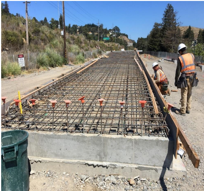
Larkspur Station Platform Ramp Construction
