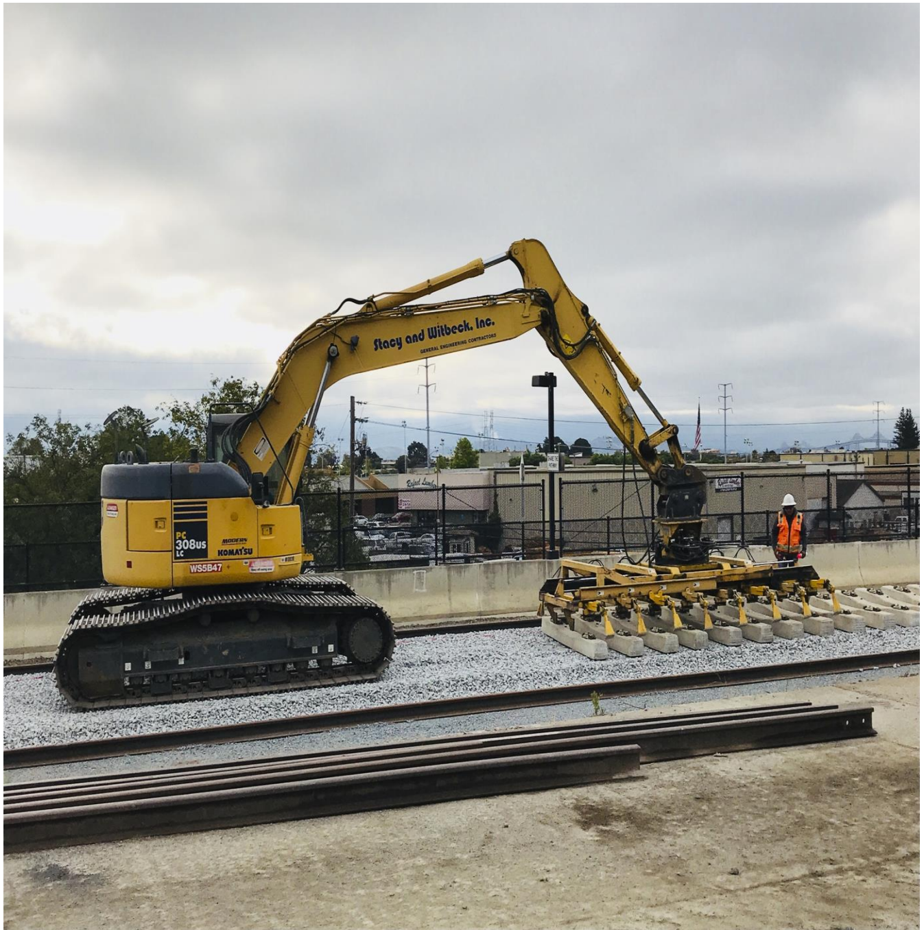
Distribute trackwork ties between the Cal Park Tunnel and Auburn Street
