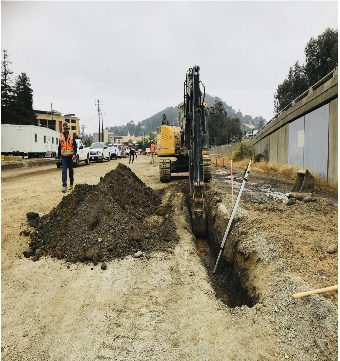
Excavation for the conduit installation
